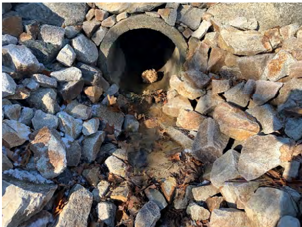
64 Gundalow - 1 (Drainage Course)
