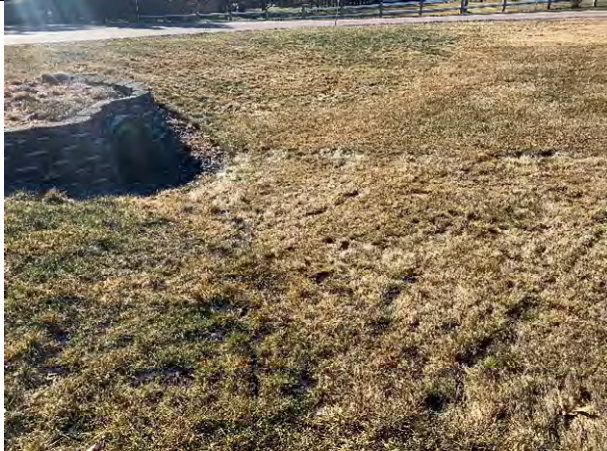
29 Gundalow - 1 (Drainage Area)
