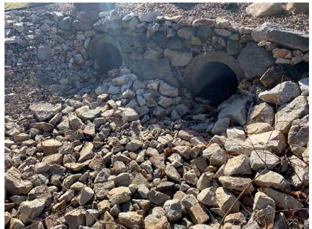
64 Gundalow - 2 (Drainage Course)
