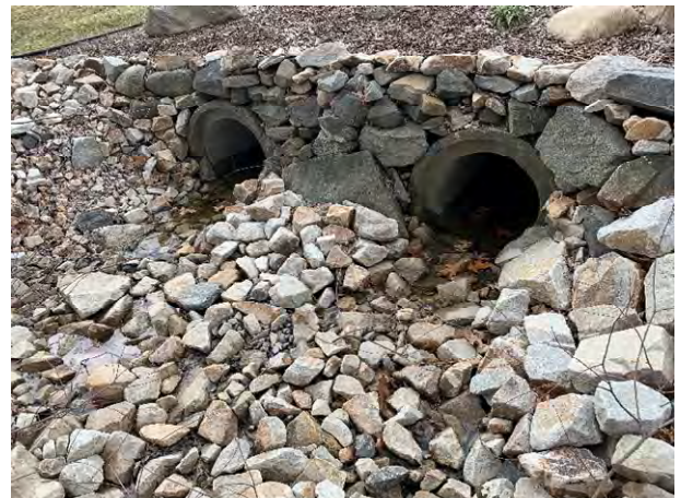
64 Gundalow - 2 (Drainage Course)
